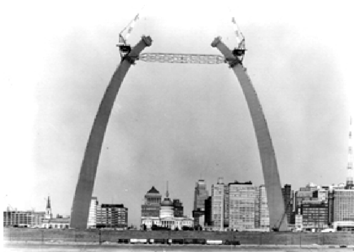
Figure 11 St. Louis gateway arch with sacrificial truss
